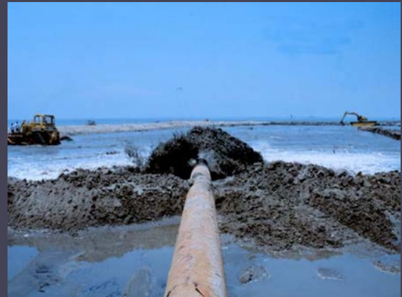
Pipe delivering sediment
